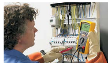
Insulation test at a distribution panel
